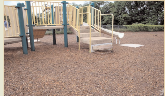
The Woodcarpet has remained firm, level and accessible even after heavy rain...
