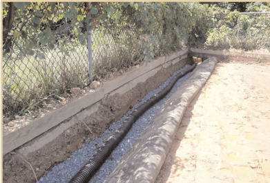
Drainage ditch and pipe installed at low end.
