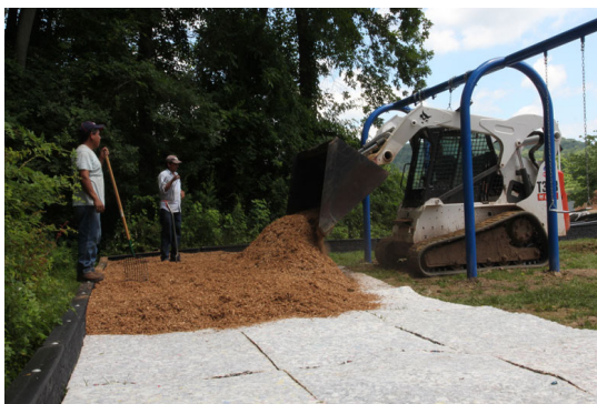
Installing the Woodcarpet over the Duradrain
