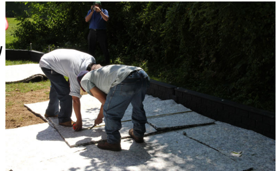
Installing the Duradrain panels.
