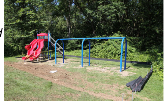
Playground equipment with borders being installed.
