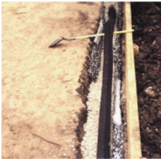
Pipe installed at low end
