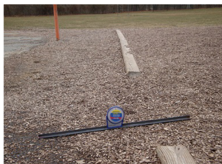
Natural ramp - opening in border
