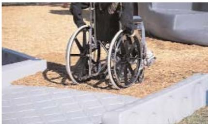
3. At accessible entrances onto the playground surface, ensure that the surface material, accessible route or the top of the access ramp is within ¼" of the top of the play area border. An ADA compliant access ramp into the play area will help reduce maintenance in this area.
