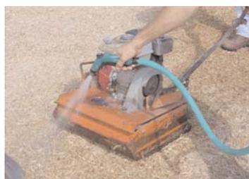
5. Once drainage is installed, proceed to install the EWF at the recommended thickness per the equipment manufacturer's recommendations. Be sure the surface is level & compacted.
