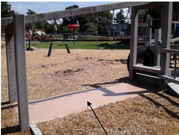
Example of a customized wear mat for an older play piece connecting entry/exit.
